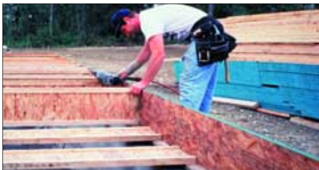
Rim board attaches to prefabricated I-joists.
