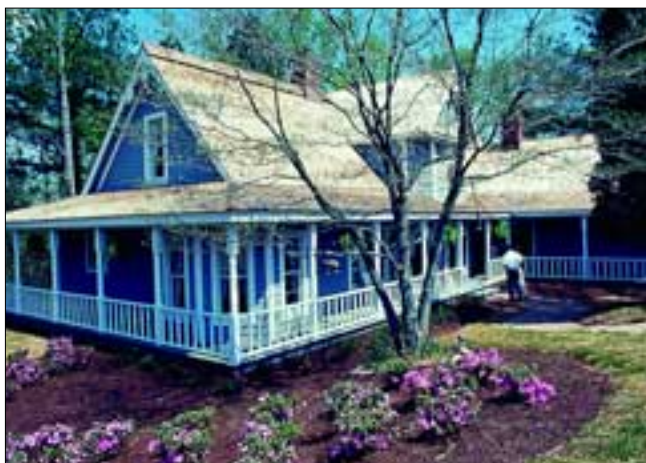
Existing trees thrive in close proximity to this pier-and-beam foundation home.
