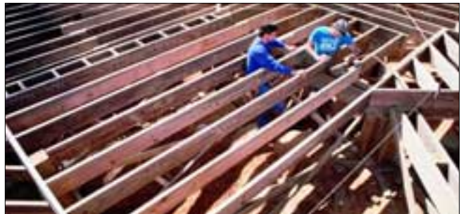
Pressure-treated Southern Pine 2x10 floor joists.
