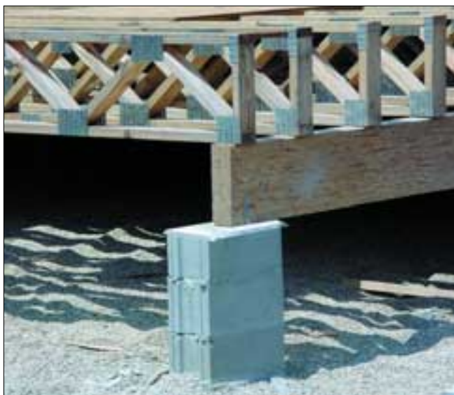
Structural composite lumber beam supports floor trusses.
