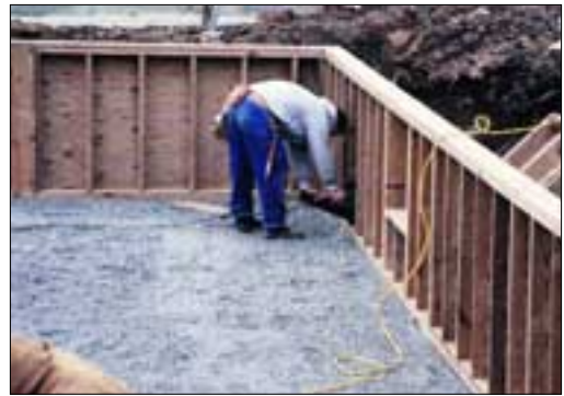
Stem wall foundations may also be constructed with pressure-treated wood members, commonly referred to as a Permanent Wood Foundation, or PWF.
